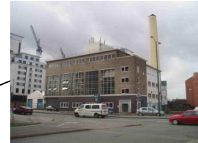
Enviroenergy District Heating plant
