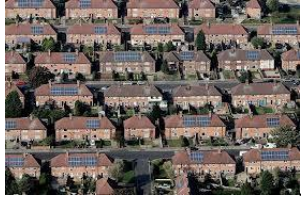
Aspley –Community "Energy Power Plant"
