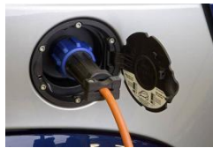
Public Charging Infrastructure
